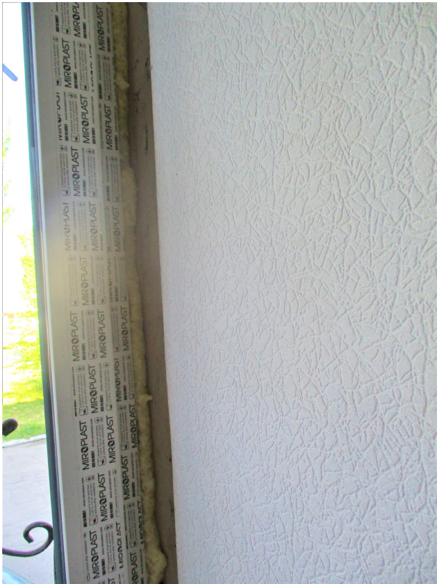
New window installed with modern spray foam insulation.
