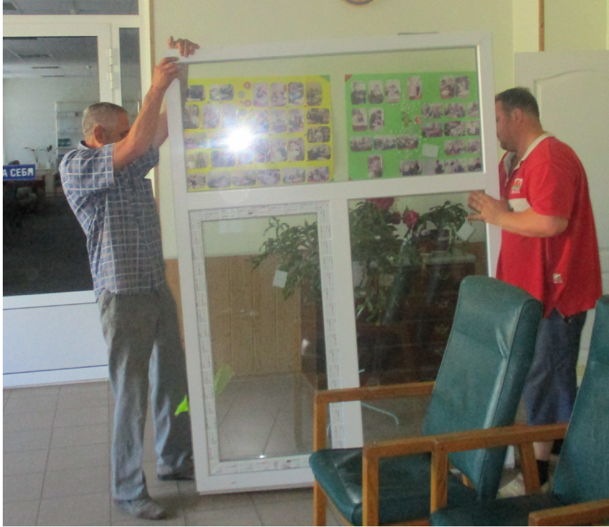
Prepping the new windows
